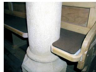
**Attention:** The "carlo" Thermodom seat heaters do not have an overheat limit device. Therefore, they must not be constantly covered. Non-observance would cause a build-up of heat - risk of fire! Unsupervised use is not permitted.
